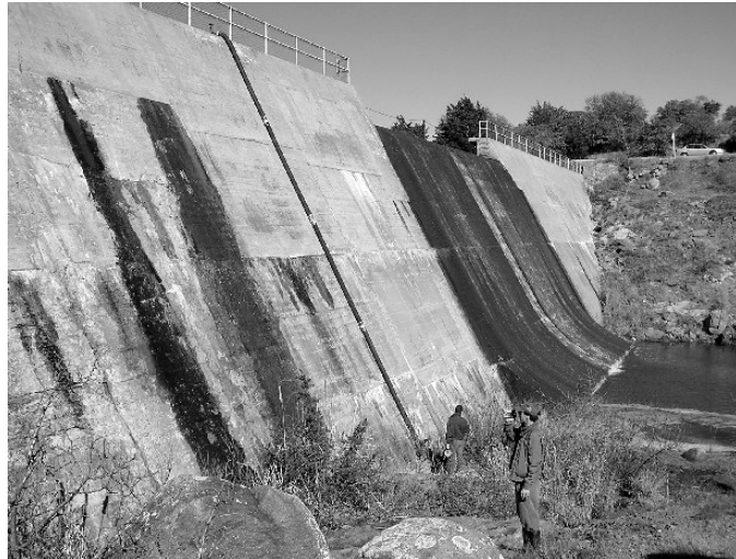
Dam Inspection at Lake Rush Dam, Wichita Mountains Wildlife Refuge, Oklahoma
